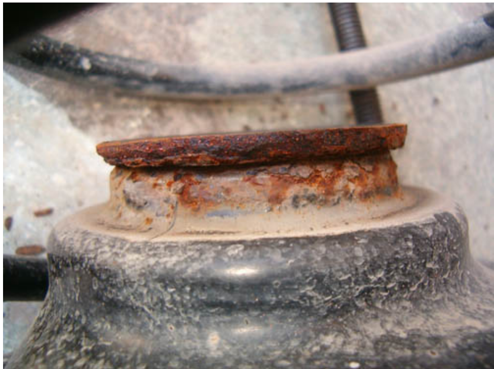
... and lower spring plate rusting away
