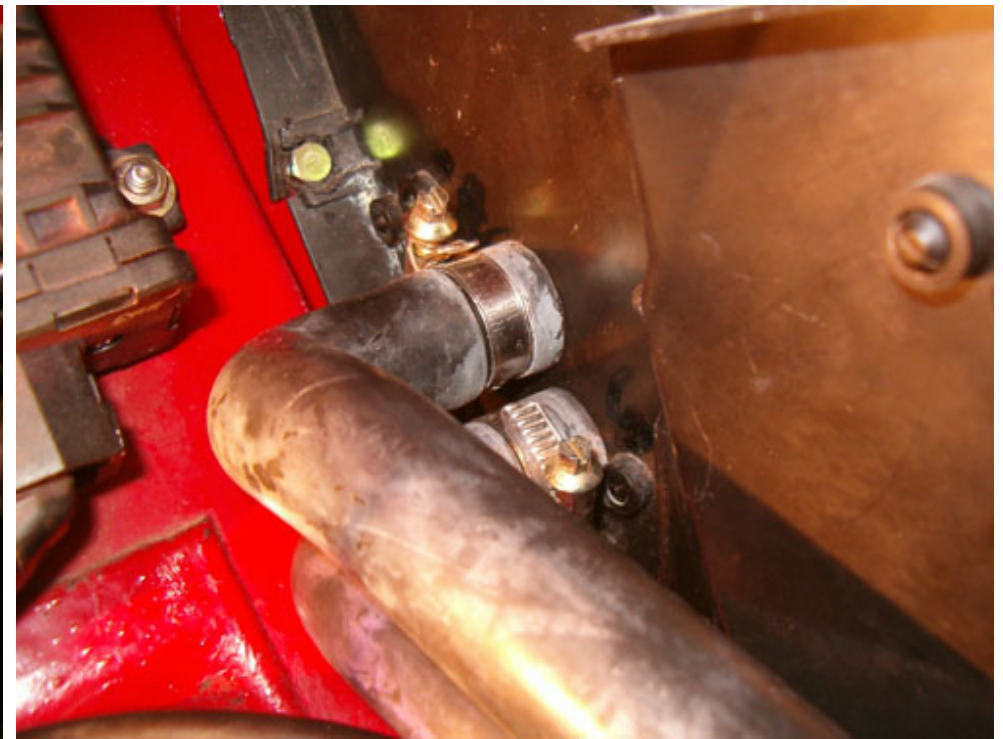
Restore heater core supply hoses ...
