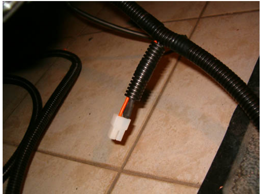
... and the first connector goes to the left condenser fan.
