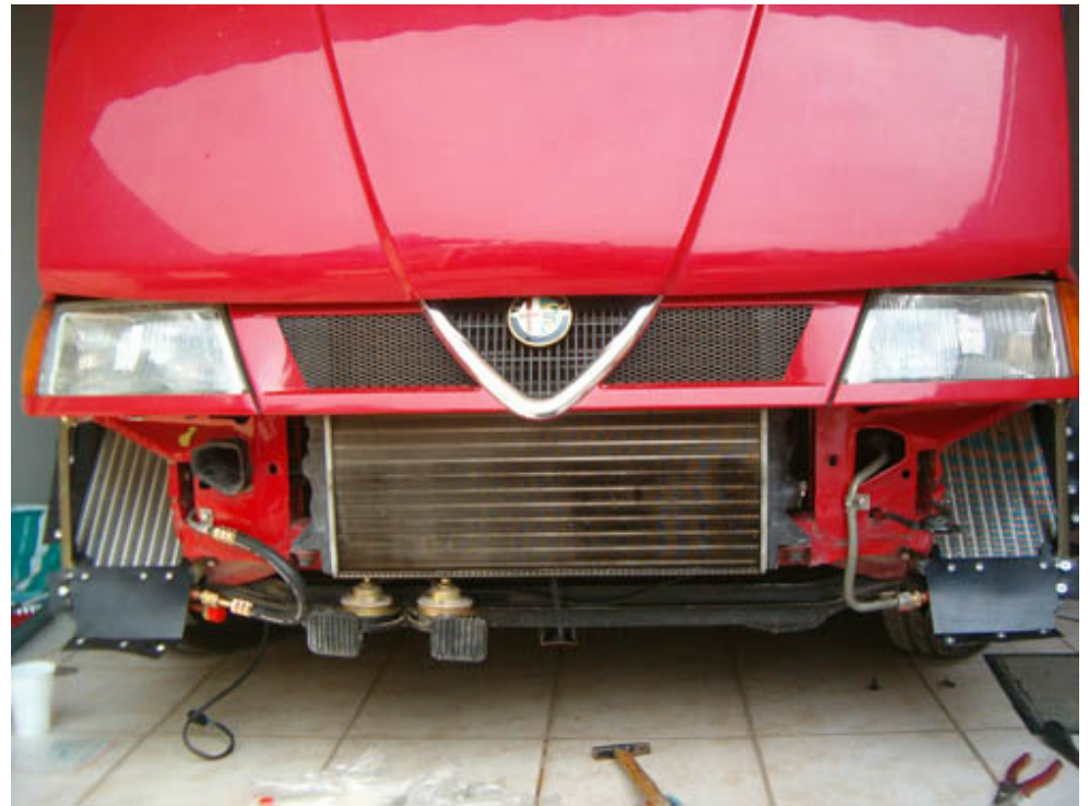
Condensers are now secured in place; let's now install Freon hose connecting them
