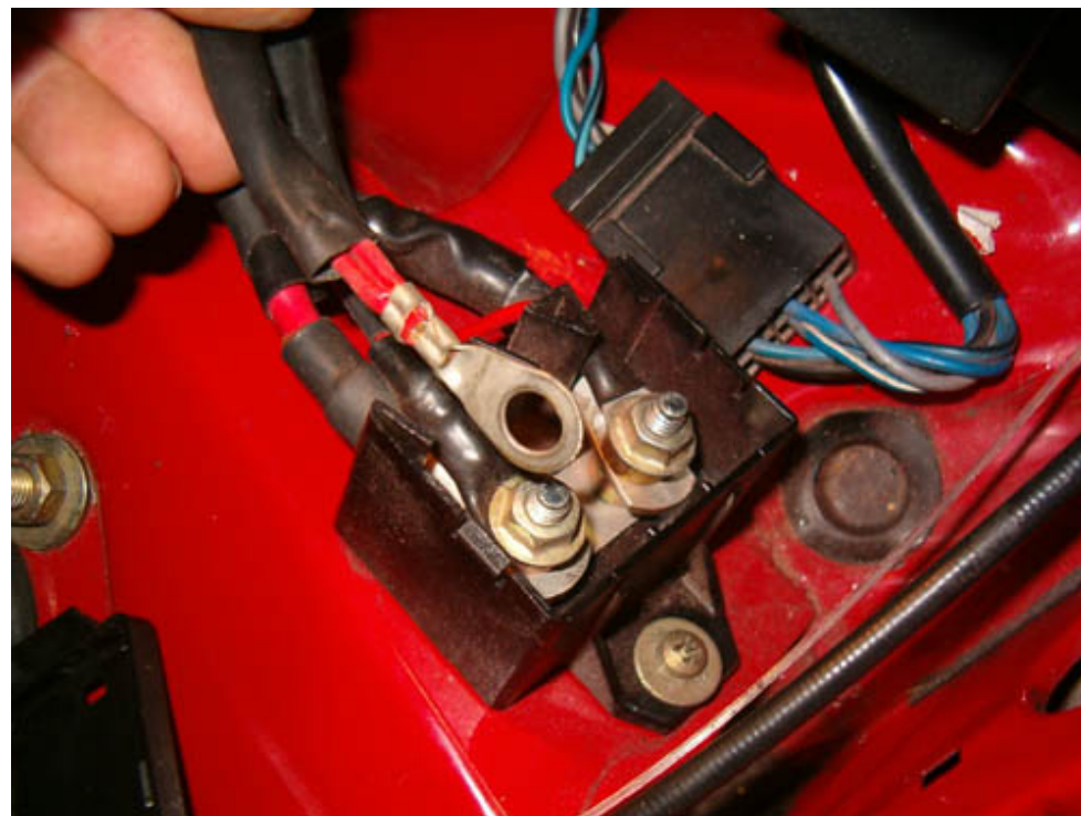
... and the positive current supply (+30 terminal) in the junction box
