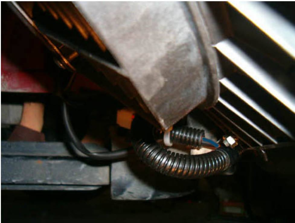
... and reaches right side condenser fan.
