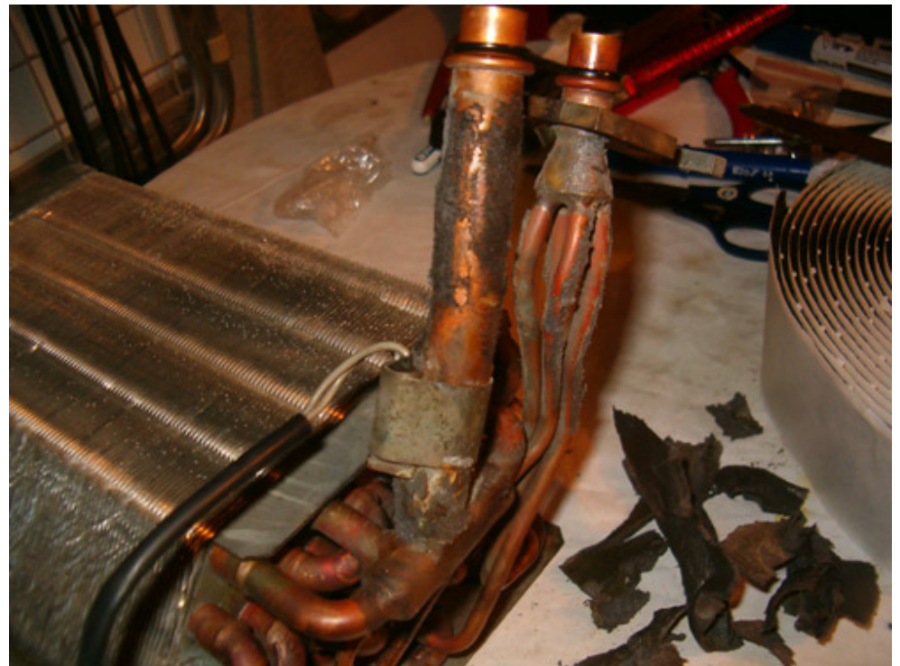
Remove the old material from the pipes ...
