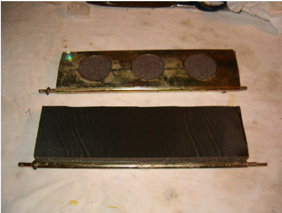
After measuring and cutting in the proper dimensions, glue the pieces together.
