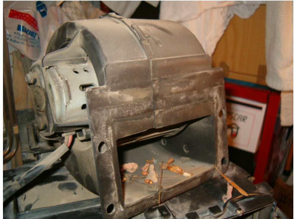
... and a hell of dirt and dust inside
