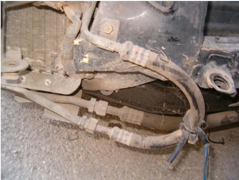
Right side condenser somehow survived from the accident but the hoses didn't so...
