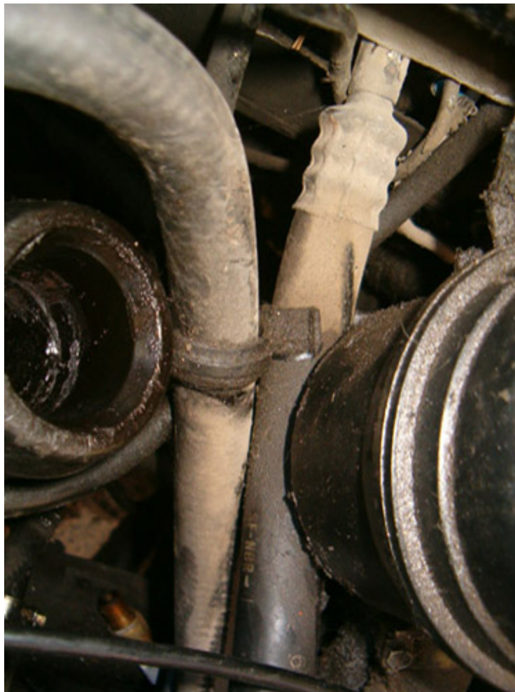
pipes leaving the firewall towards the compressor
