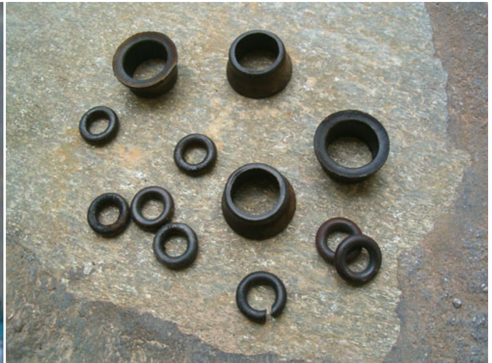
Old O-rings which will be replaced with new ones
