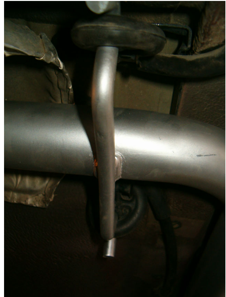
Rubber support rings are installed in place
