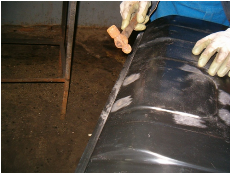
Using the rounded end of the hammer the welds are flattened, so as patches are level
