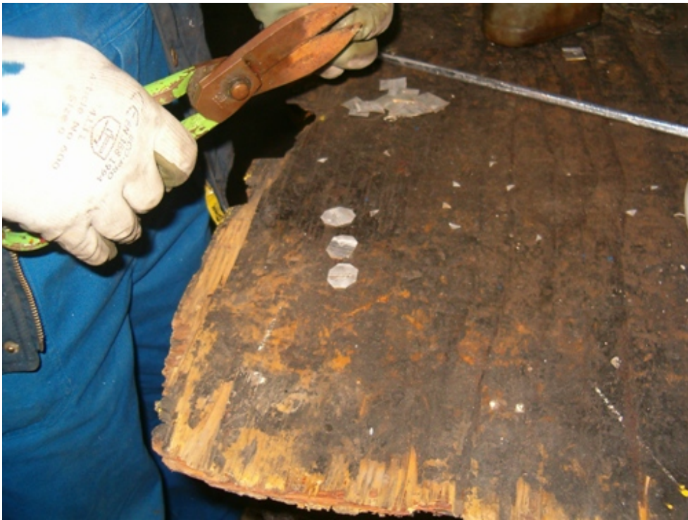
The patches are almost ready in round shape. The material used is brass in thin leafs.
