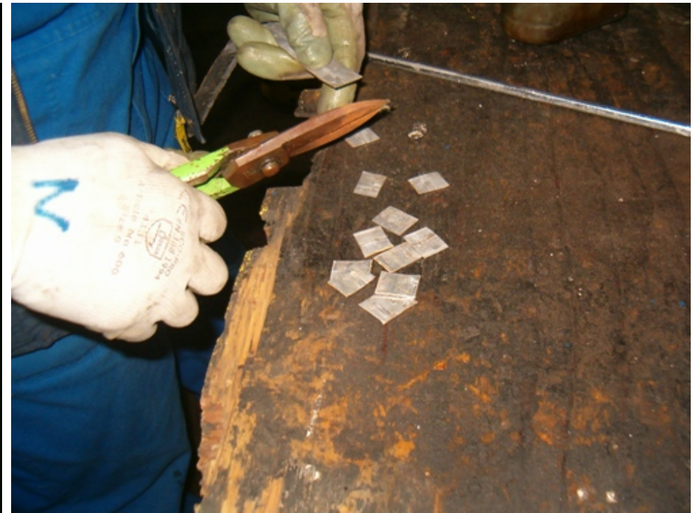
Here you can see the patches being prepared
