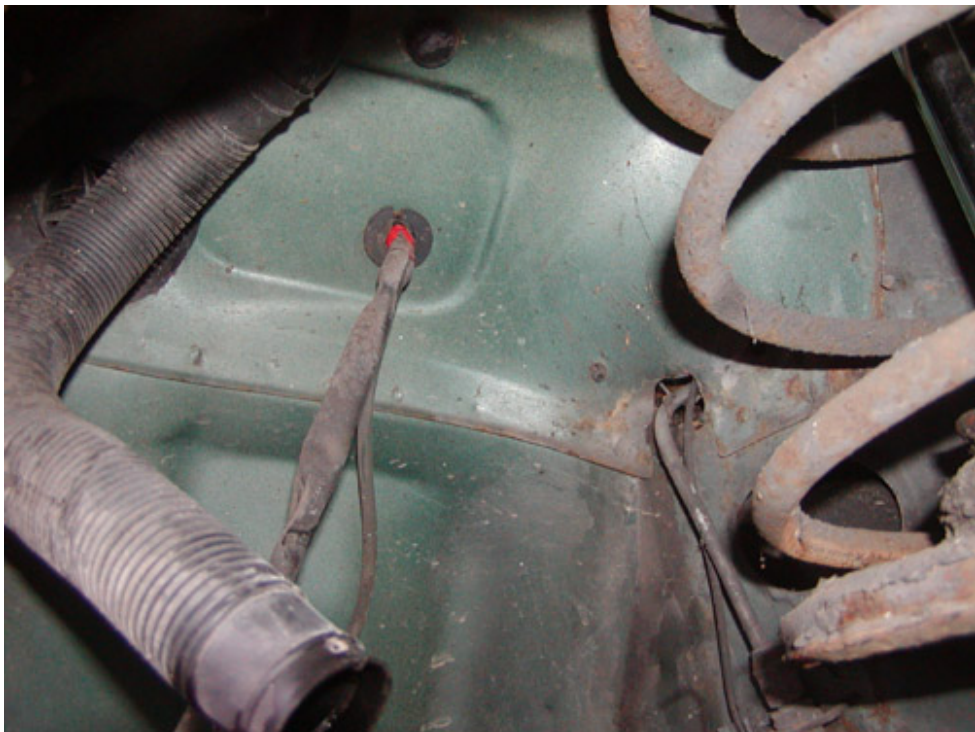
Wiring passing through the left fender well
