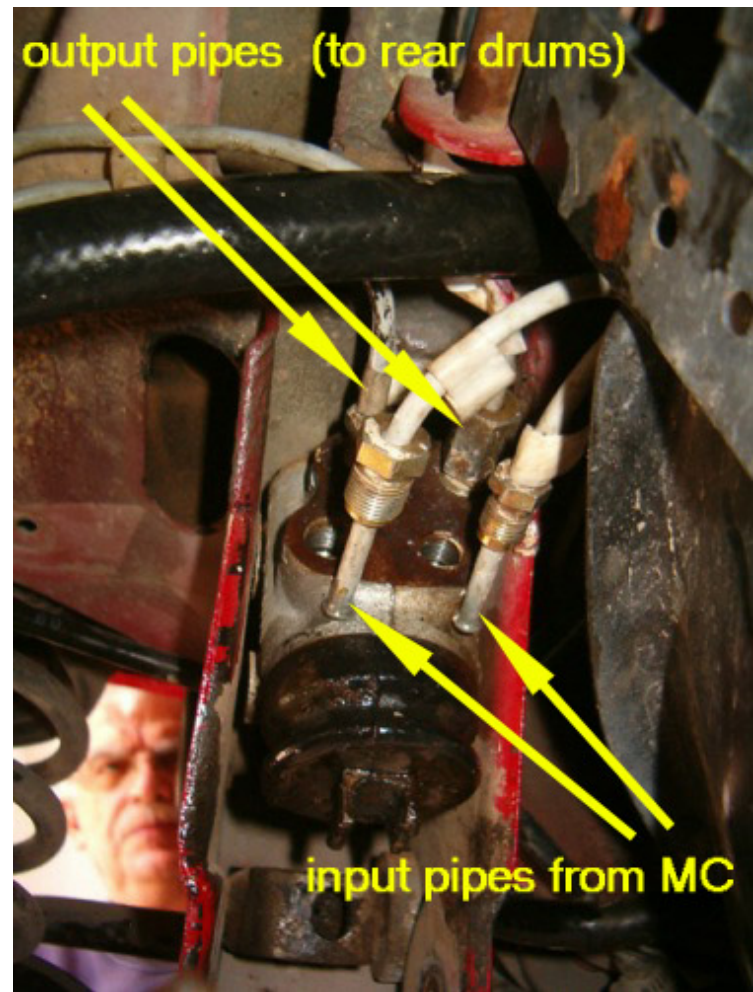
Time to remove the bias valve. It is advisable to marke the brake lines so that you don't mix them up while refitting
