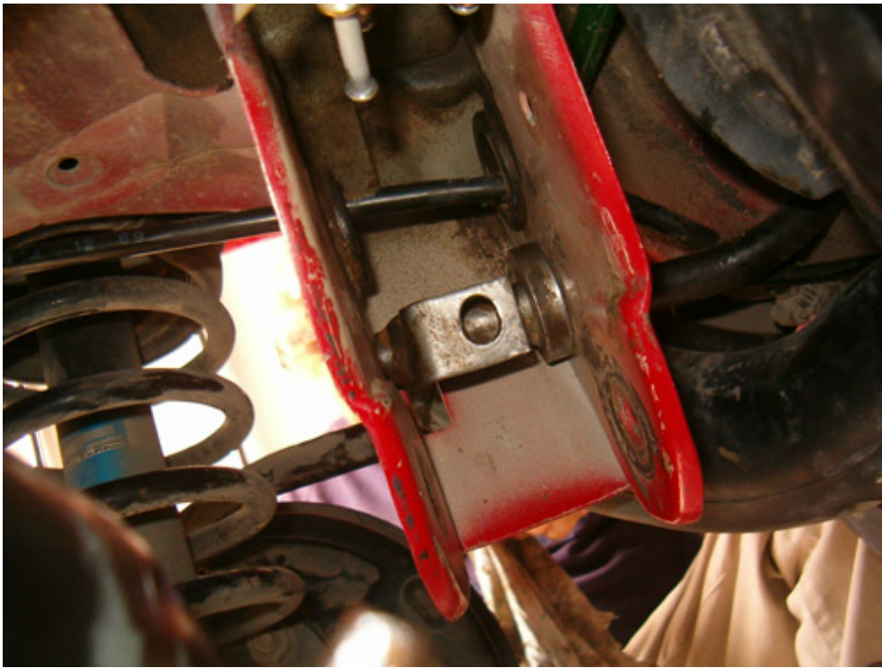
I have cleaned up the cavity and installed the adjustment hook
