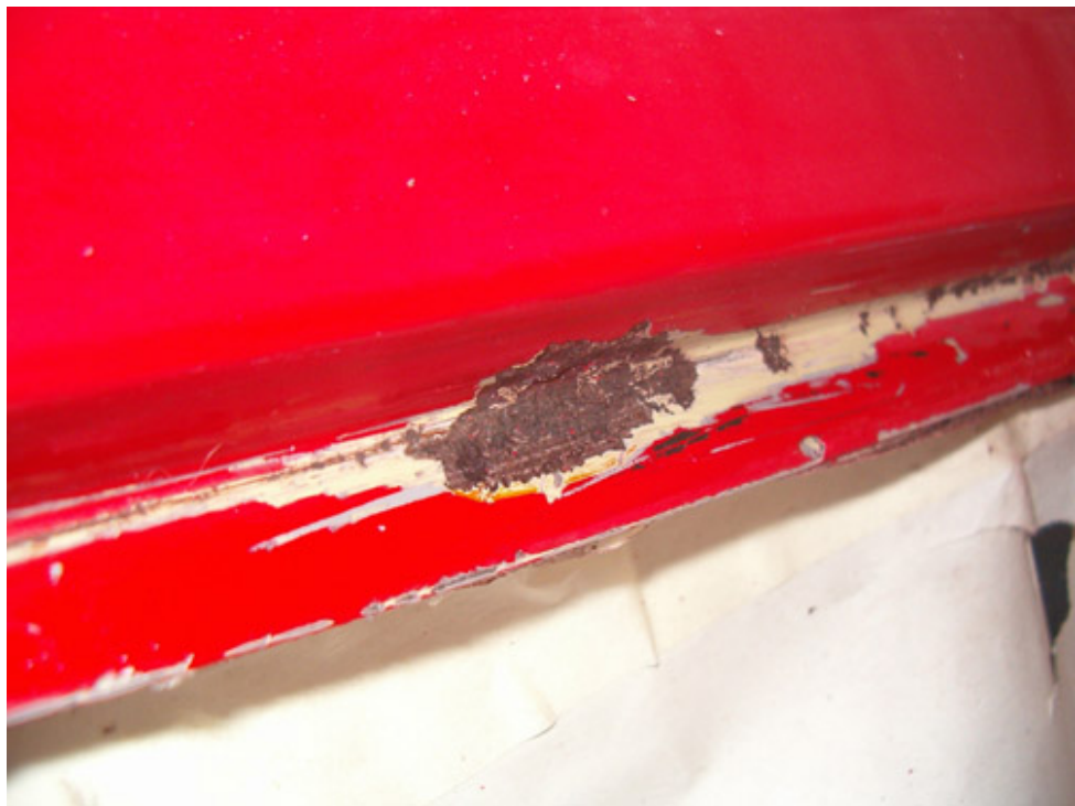
Once everything is cleaned rust spots were revealed on the upper side of the frame.
