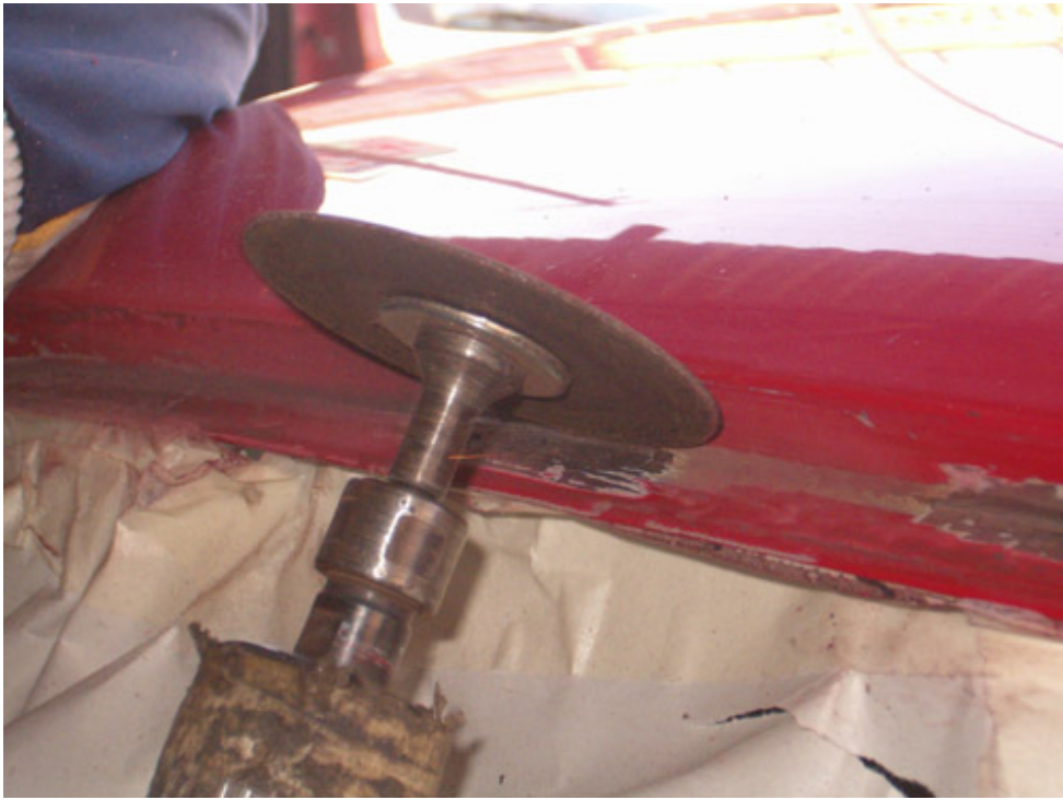
The grinder rubs rust to clean metal.
