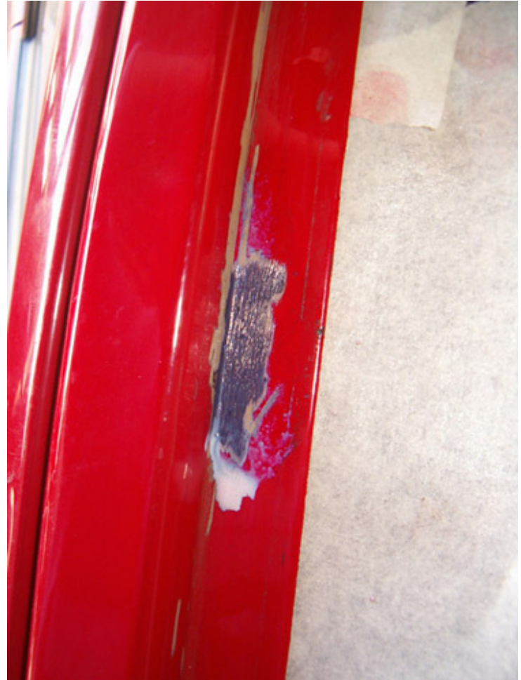
Rust inhibitor is applied once the rust spots are clean
