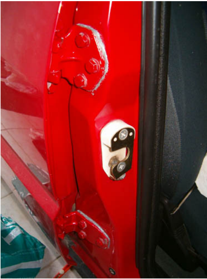
End result before painting the sealed area
