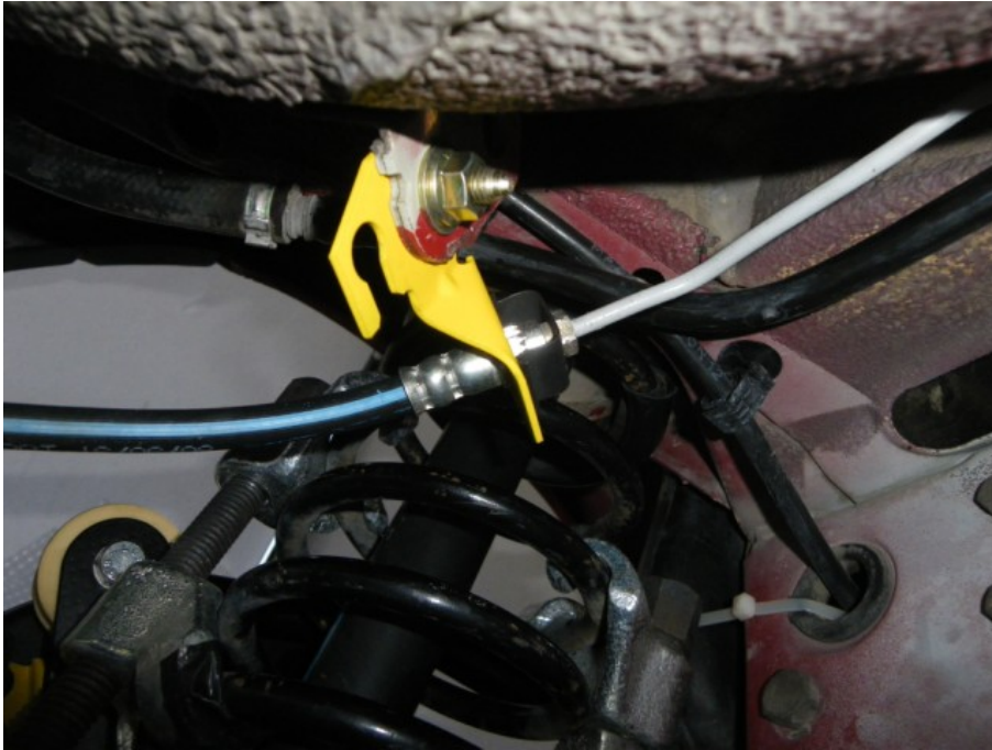
Finalize installation by fully tightening the brake line/hoses unions
